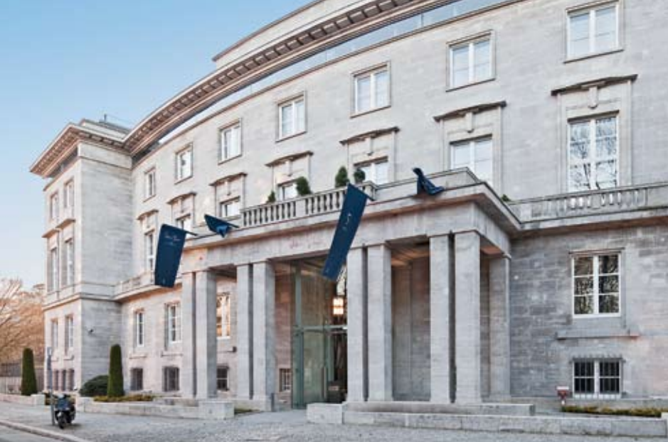
Clockwise from top left: The only modification to the landmarked 1940 limestone facade is a glassed-in entry. Custom-printed cotton covers part of the ceiling in reception, where seating is by Studio Urquiola. A guest suite's built-in headboard is cerused oak. The lobby features a bronze crocodile sculpture by Quentin Garel. A Studio Urquiola sofa in the lounge is strewn with pillows covered in wool-nylon.
